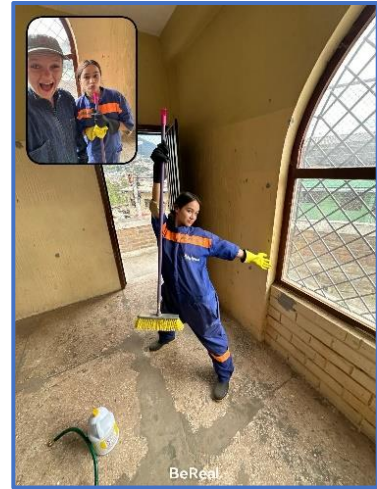
The interns cleaning before painting acting like Bob the Builder.
